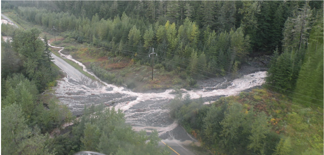
Alaska-Stewart Highway Flood of 2011. Image courtesy of B.C. Ministry of Transportation and Infrastructure
